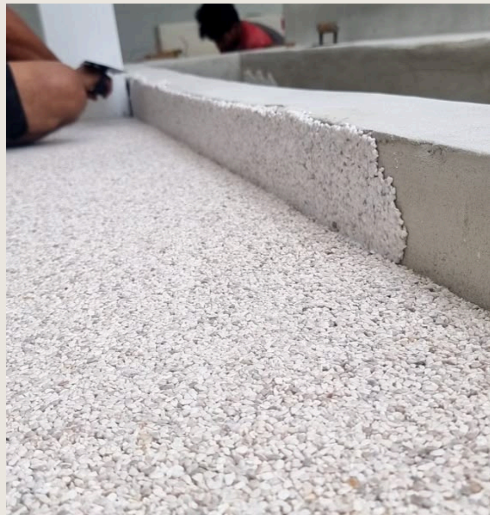
2MM GRANULES MORTER APPLICATION ( 2026)
